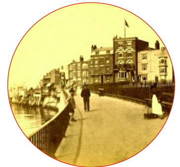
This old photograph c.1860 of Hazardous Row illustrates the importance of Andrew's Passage before Marine Drive was built in 1880
