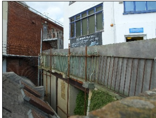
Showing the crumbling footway alongside The Sundowners' Bar
